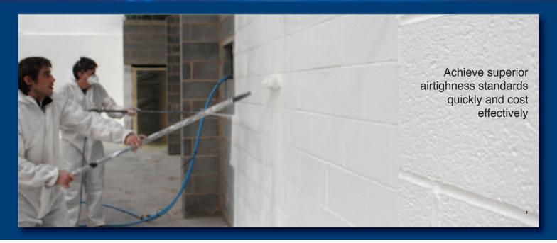
Concrete block walls can leak the air in a building at up to 80 cubic metres of air every hour through each square metre of surface, at that rate it won't take long for the air inside to escape from the building, resulting in increased heating costs & carbon emissions
